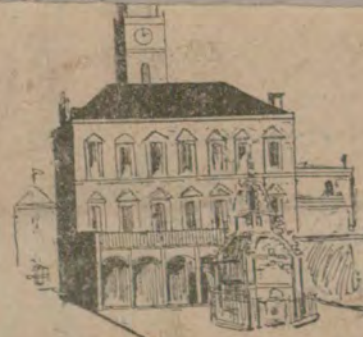
The above is a sketch of the Linlithgow Old Tolbooth, which is at present the subject of dispute between the County Council and the Town Council of Linlithgow. The old jail consists of the basement
