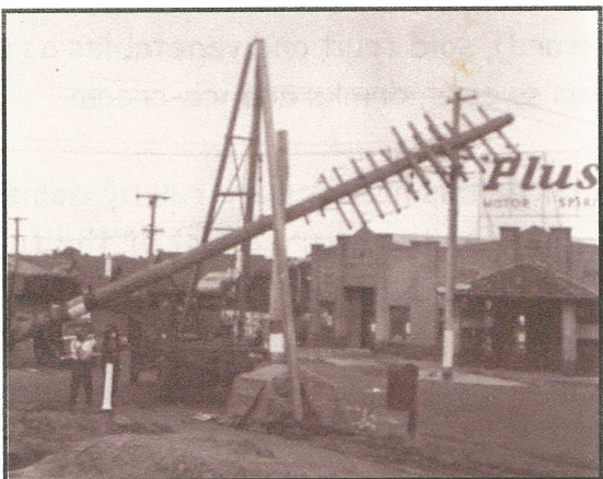
Circa 1930: Installing a new power pole, to upgrade the electricity in Bentleigh. Site is the corner of Centre and Jasper Roads. J L Smith's garage in the background. (Safeway's today)
