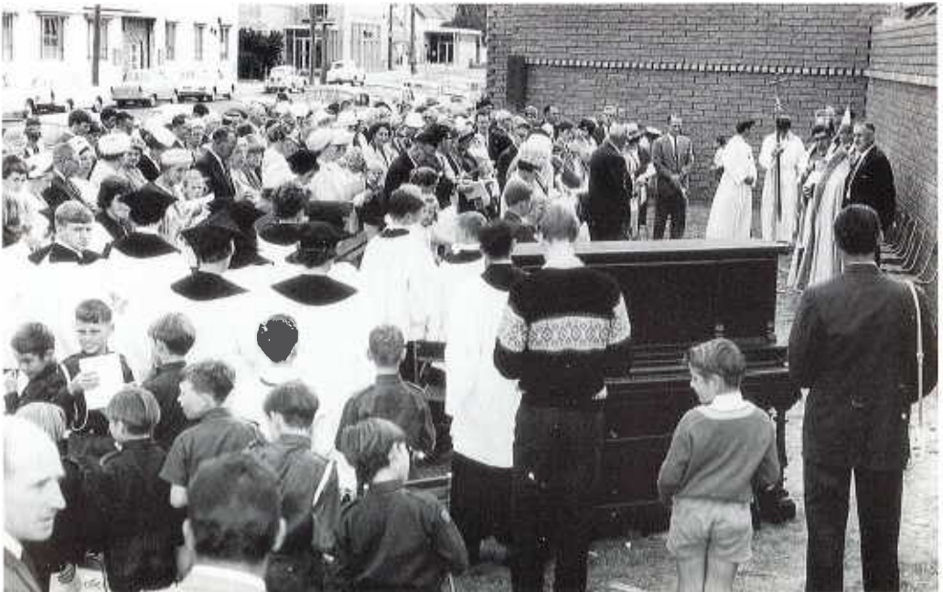
Setting of Foundation Stone by Bishop Amott, March 1966 (ref. p33)
