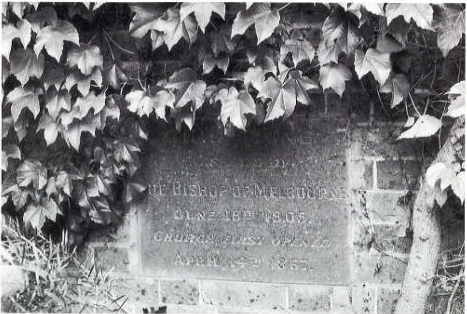
Foundation stone of Chancel (ref. p13)
