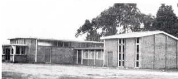
The new St Francis'
