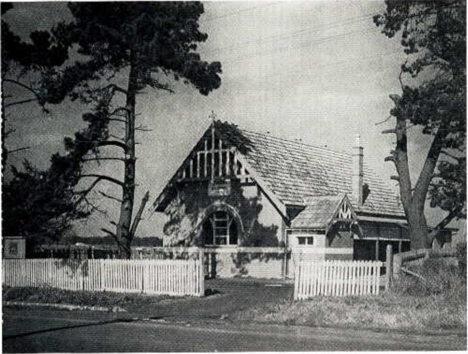
1940 and still surrounded by market gardens — the old brick school in Centre Road.
