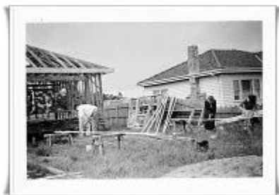
Installing the weatherboards (Chapman Street, Macleod - 1956)
