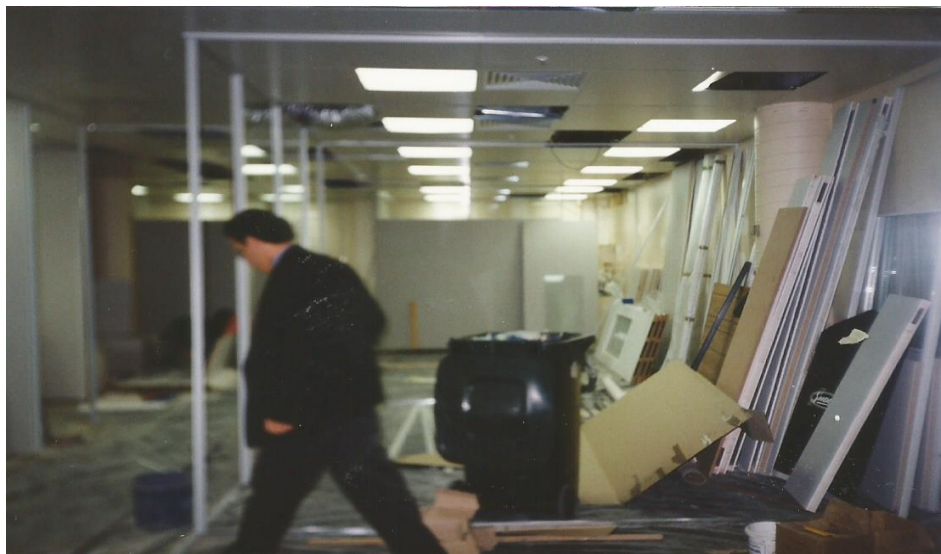
Shop renovations in progress at shop 201. 1996. (Pictured above).
