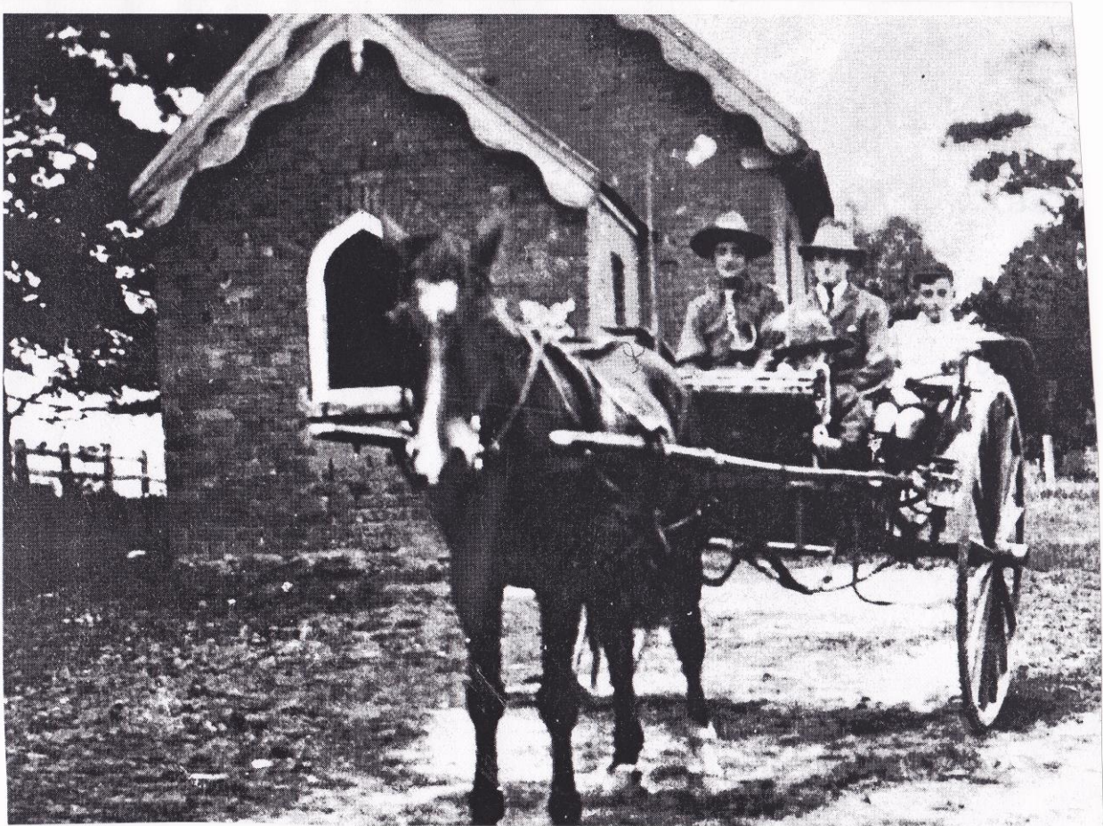
Old Anglican Church School (No. 268), built 1855. Photo about early 1920s.
