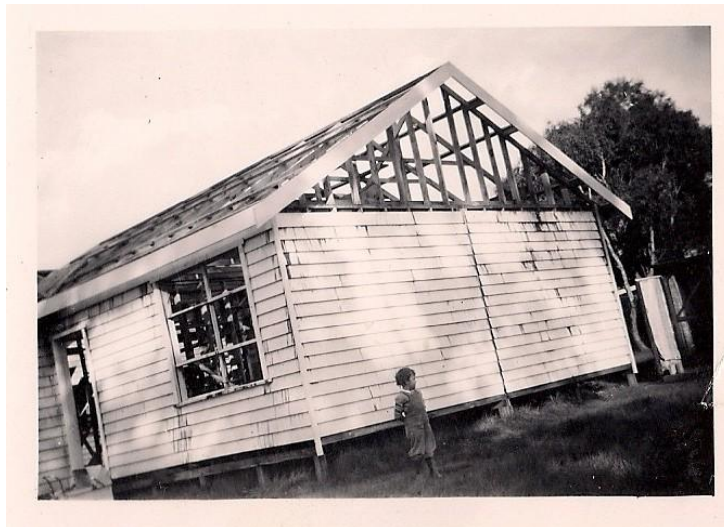
2. No roof and no chimney
