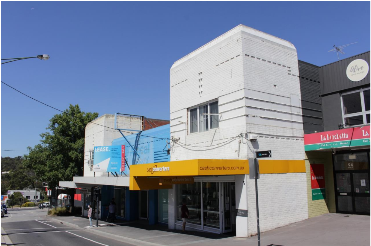
Stubleys viewed from the west
