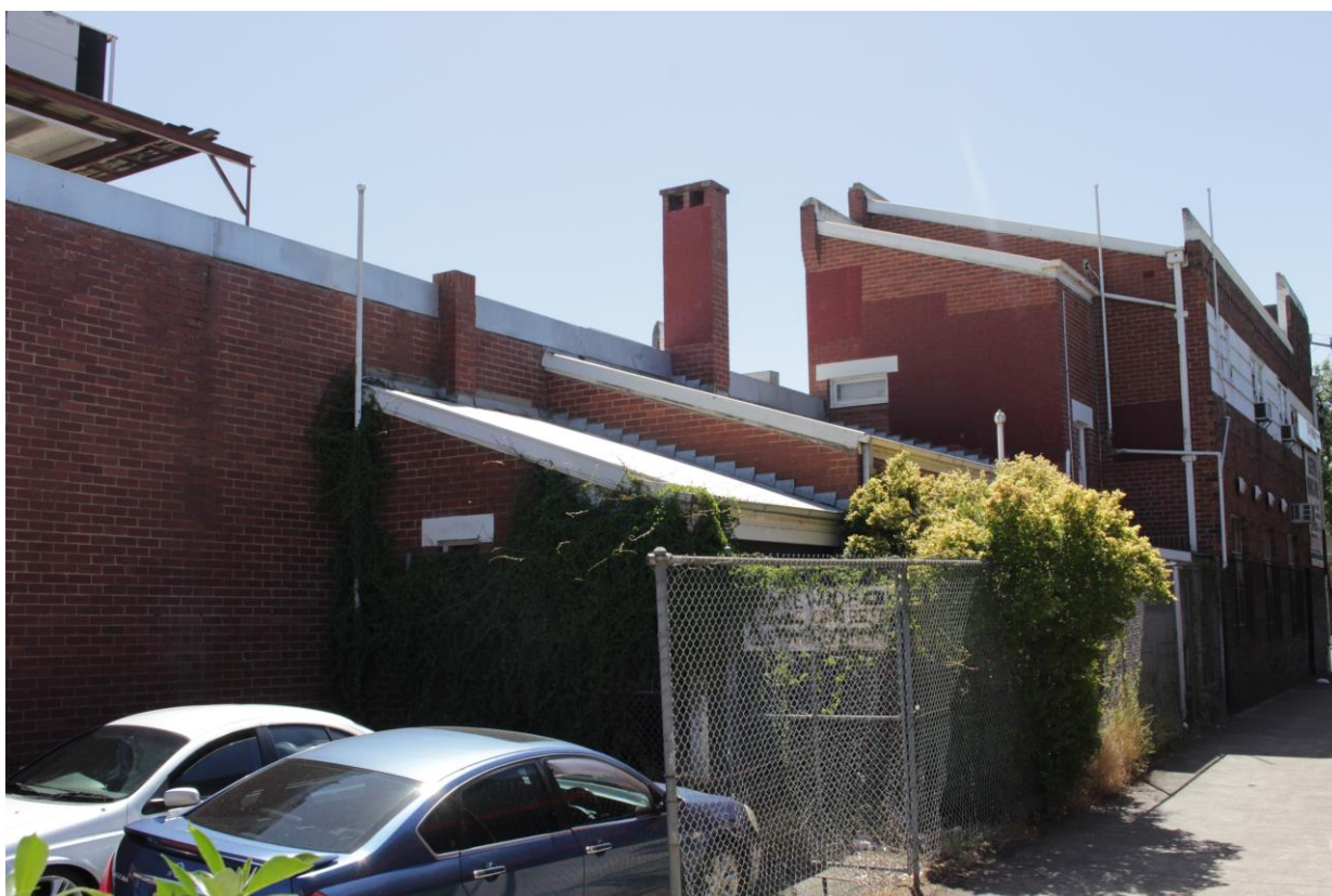
Lean-to volumes – east elevation, facing north
