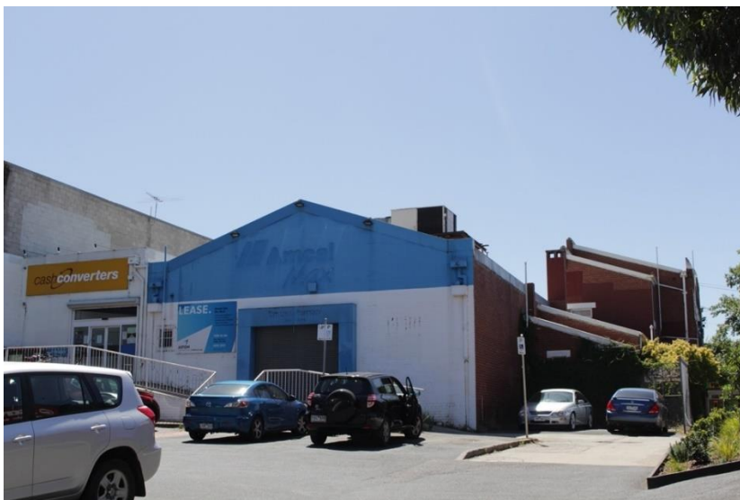
Rear – later addition wing is left of frame
