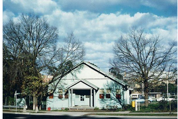
Photograph of the Greensborough Park Tearooms from Diamond Valley Creek Road, in 1978, prior to additions (Source: wikinorthia)
