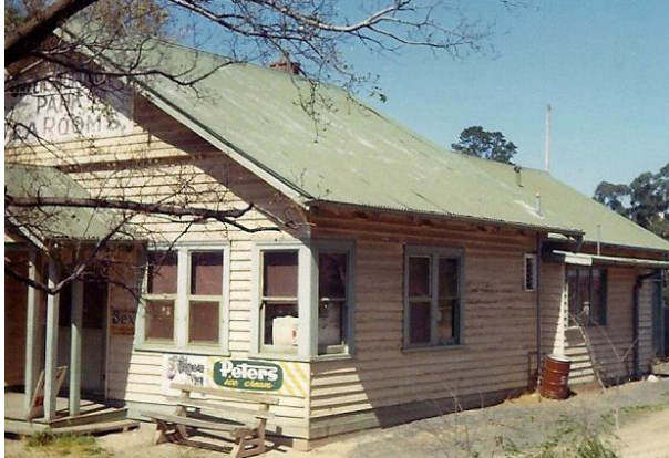
Photograph of the façade (left of frame) and northern elevation in the early 1960s (Source: courtesy of Greensborough Historical Society)
