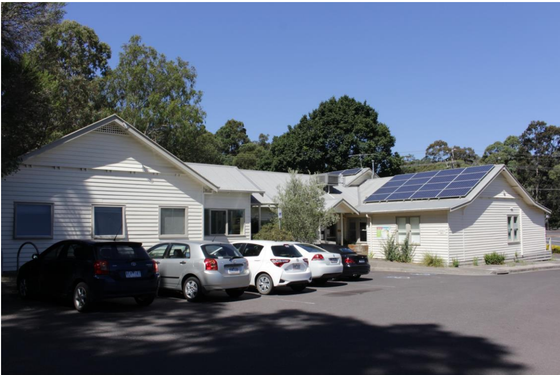
View to later additions from the rear carpark – the former tearoom is situated right of frame
