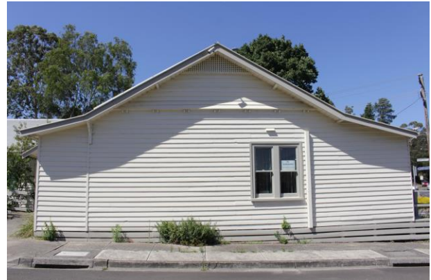
1925 rear – flanking skillion volumes are later additions
