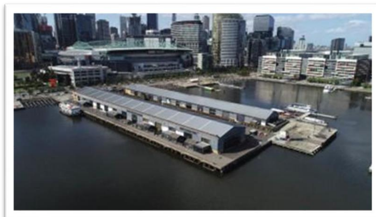
Figure 5: Photograph of Central Pier at Docklands
