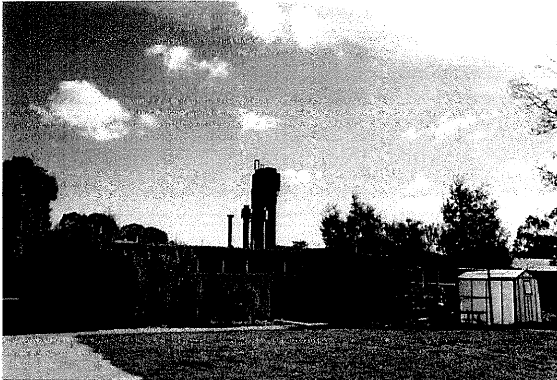
Ringwood Secondary College - Bedford Road (north-west corner of Hill Street), Ringwood
