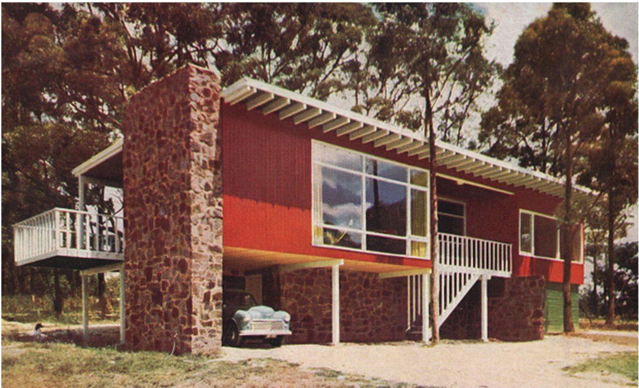
Photograph of the Kotzman Residence soon after completion, 1954 (Source: Kenneth McDonald, The New Australian Home )
