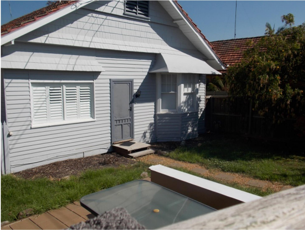
House at No 1/110 Bedford Road
