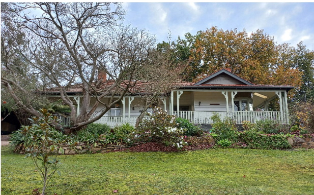
Former private hospital at 16 Ellesmere Avenue (1923)
