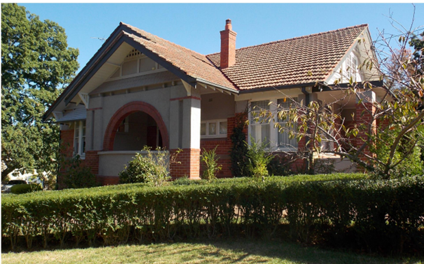
Brick and roughcast villa at 23 Alto Avenue (1923)
