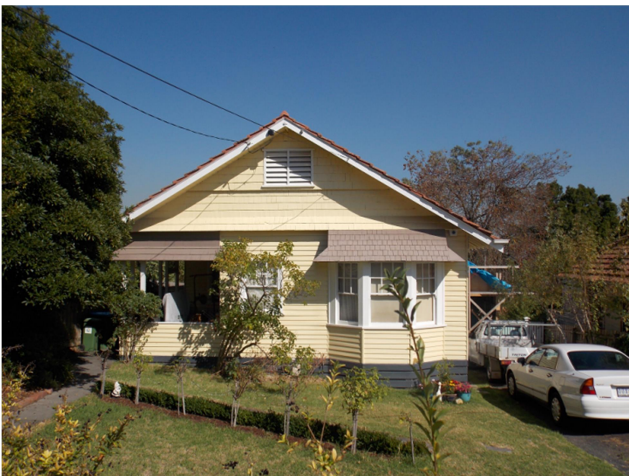
House at No 124 Bedford Road
