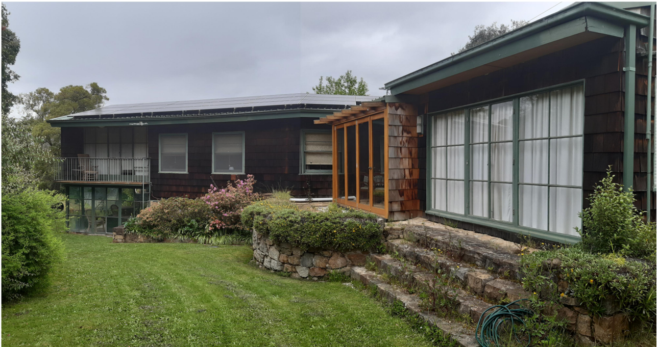
Composite panoramic photograph of the Heathmont Road frontage, taken by City of Maroondah, October 2020 Note stone terrace, steel-framed window wall to living room (right), projecting sunroom with timber-framed glazed doors, and master bedroom wing (far left) with another steel-framed window wall, balcony and glazed infill below.
