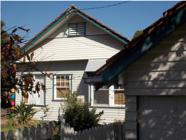
House at No 120 Bedford Road
