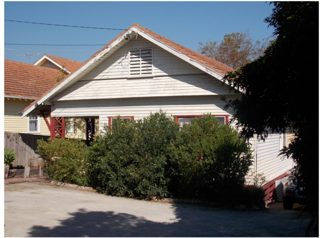
House at No 122 Bedford Road
