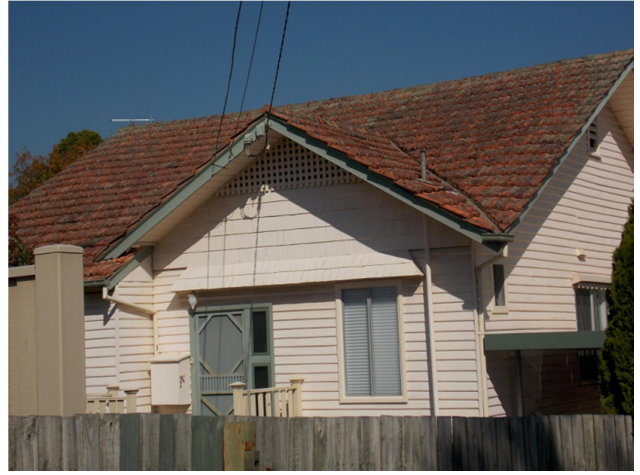
House at No 116 Bedford Road
