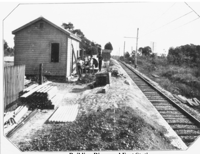
Building Ringwood East Station
