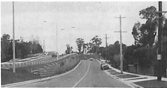
Duplication of road pavement in Canterbury Road.
