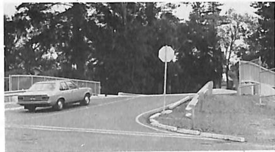
Reconstructed Eastfield Road Railway Bridge.
