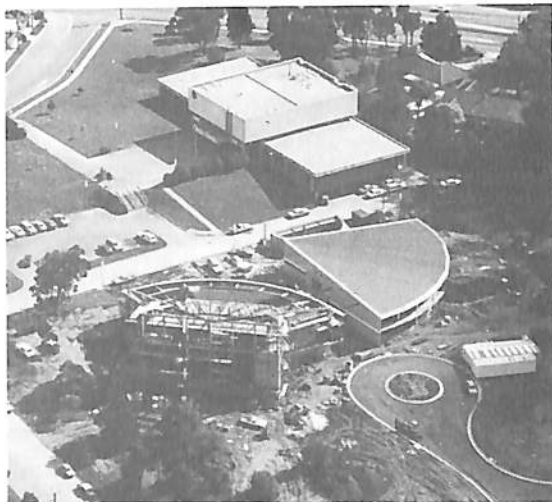
Ringwood Civic Centre featuring Stage 2 under construction
