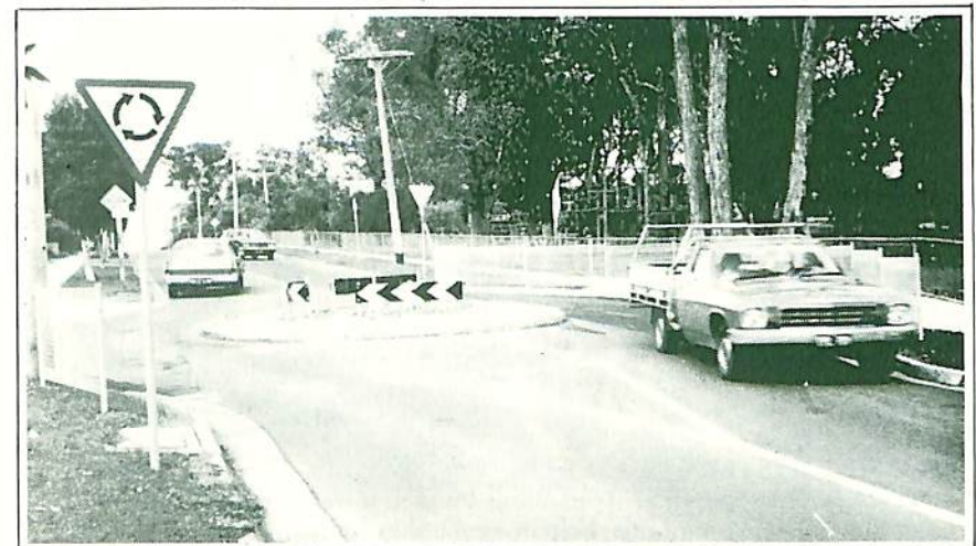
Traffic management experimentation in conjunction with the Road Safety and Traffic Authority in Maidstone Street.
