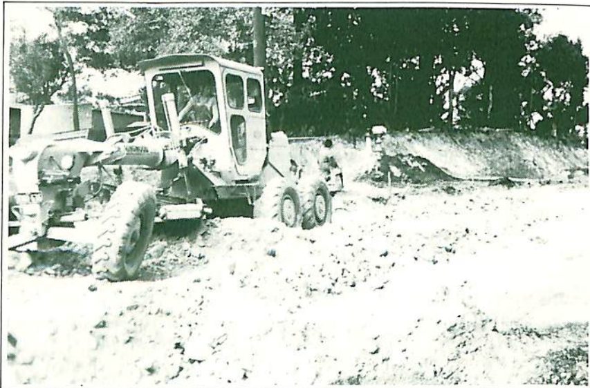
Glenvale Road under construction north of Kubba Road.
