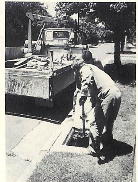
Council employees clearing debris from a drainage pit
