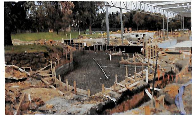
CONSTRUCTION OF THREE DEPTH TODDLERS POOL
