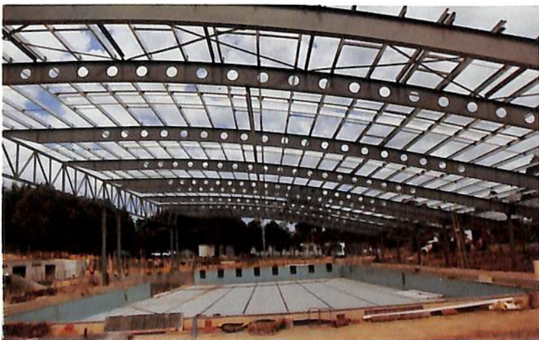
ROOFING OF EXISTING POOL
