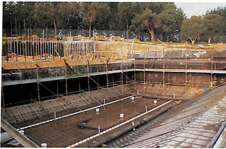
CONSTRUCTION OF DIVING TANK
