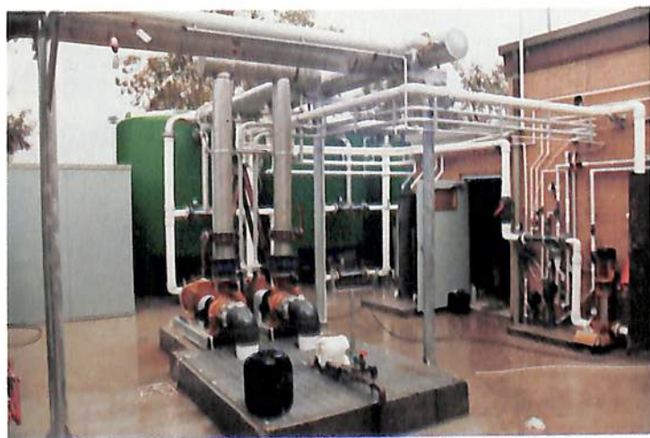
OZONEATED, FILTRATION AND DE OZONEATED PLANT
