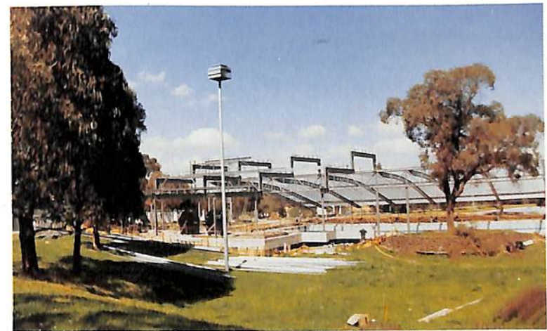
VIEW OF MAIN POOL, EXTENSION AND ROOF CONSTRUCTION
