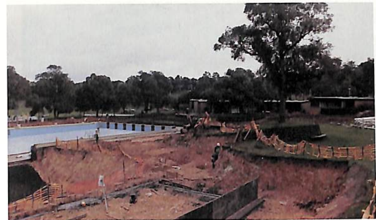
INITIAL SITE WORKS IN PREPARATION FOR CONSTRUCTION
