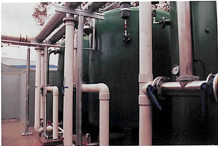
OZONE TREATMENT TANKS
