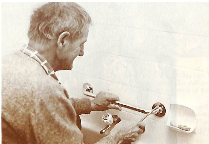
Home Handyman Chick Smith fitting a handrail
