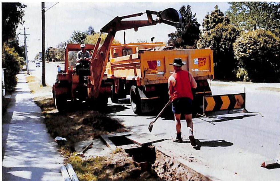
Drainage works in Wantirna Road
