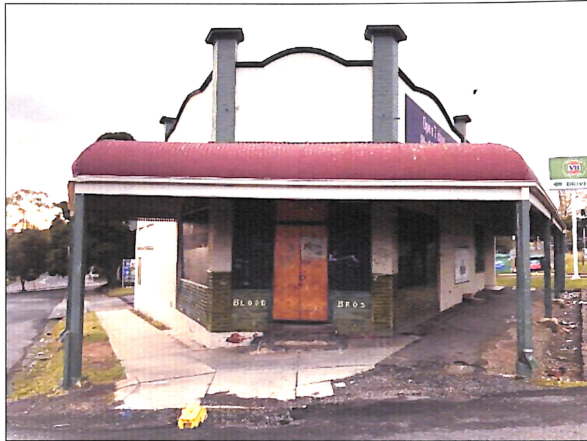
Figure 20 View of the western corner return showing the main entry to the shop, with the encircling reproduction verandahs along its Station Street elevation (left) and Bedford Street (right).
