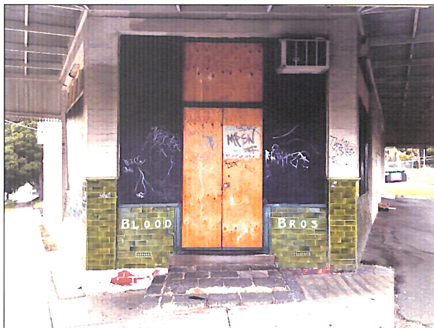
Figure 21 The shop front to the main entry includes green glazed tile dados. Doorways and windows have been boarded up.
