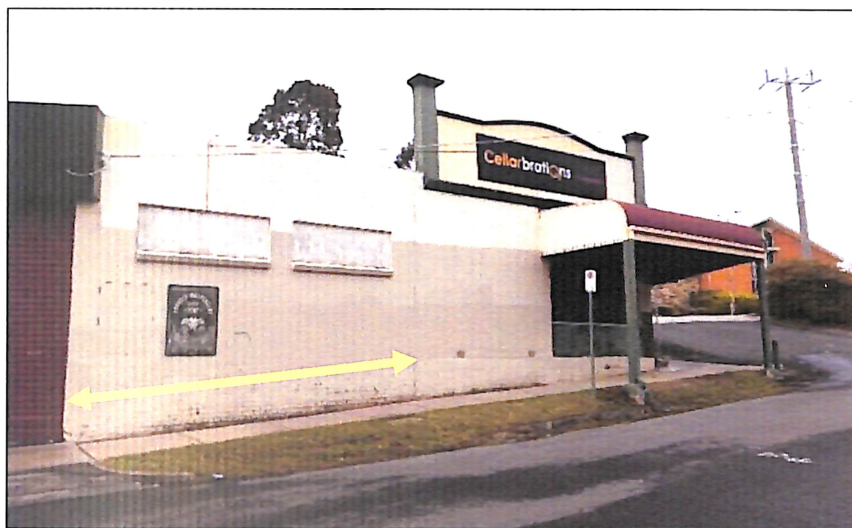
Figure 29 The north elevation of the shop to Station Street, showing the remaining original portion of the shop with the high parapet at right, with the extent of the eastern c.1980s brick addition indicated by the yellow arrow.
