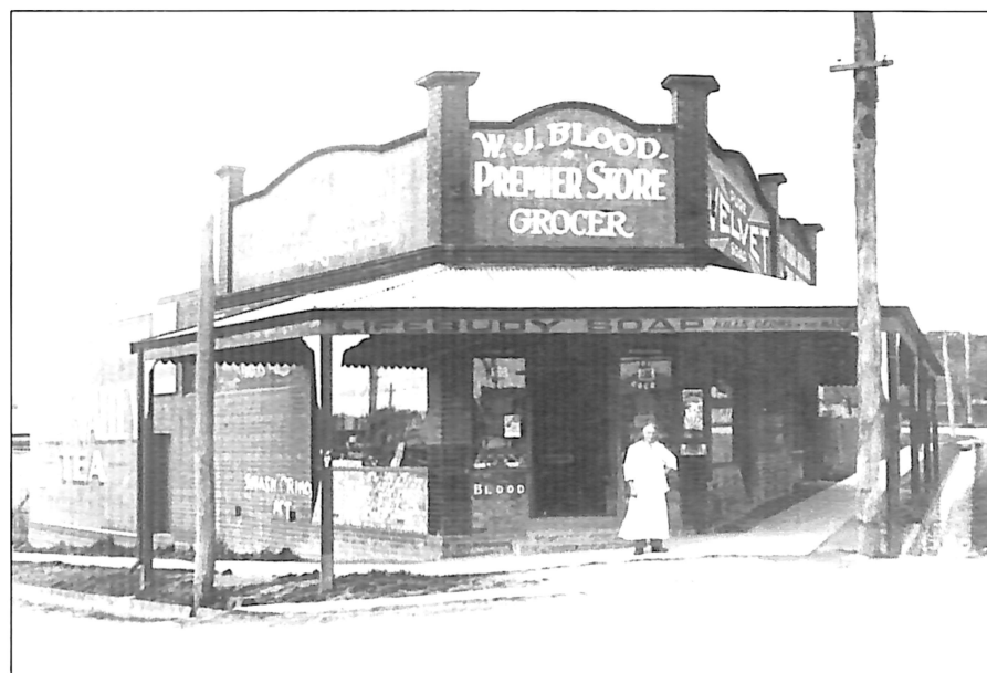
Figure 11 c.1924 image of the store showing more of the north elevation (left) with William (Bill) Blood by the front door. Source: Ringwood & District Historical Society.
