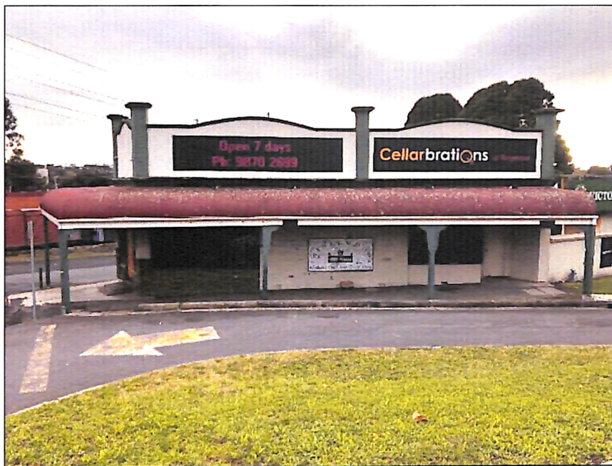
Figure 23 The south elevation to the original portion of the shop facing Bedford Road, showing the extent of the reconstructed verandah.
