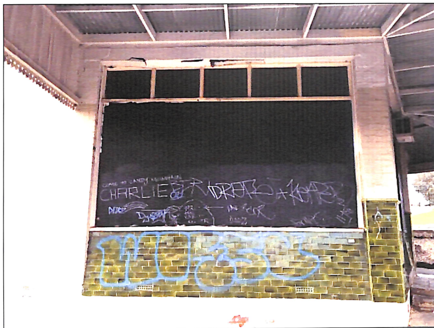
Figure 27 The shopfront to the northern (Station Street) elevation, showing the glazed dado tiling and simple window form.
