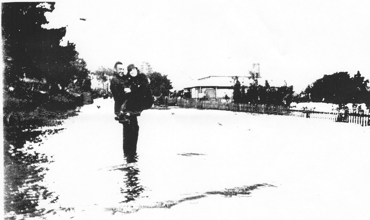
Looking west along Yarra Street from Whipstick Gully with Bishop's house in the central foreground, this photo shows the 1934 flood in Warrandyte. At the time the photo was taken the floods are probably receding, as when floodwaters peaked the fence was completely covered. The names of the man and woman are not known but any details are welcome.
