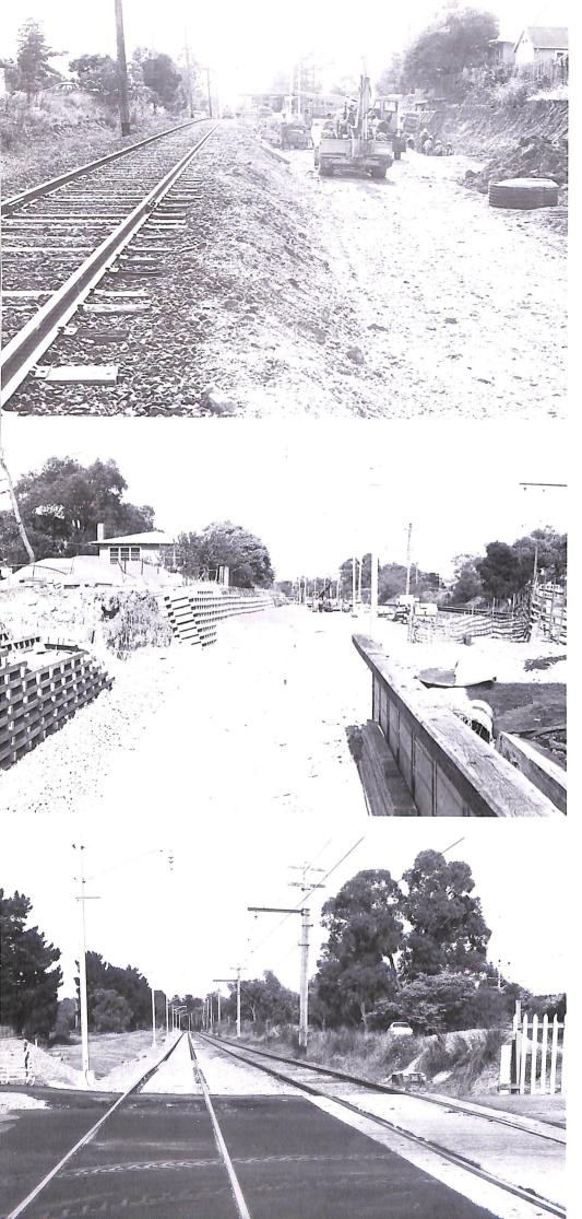
Three views of the Ringwood to Croydon duplication project. (Top) The groundwork for the construction of the second track is carried out on the far side of East Ringwood Station. (Centre) A different view from the Station of the same work. (Below) The double track has already been laid at the Dublin Street level crossing down from the Station
