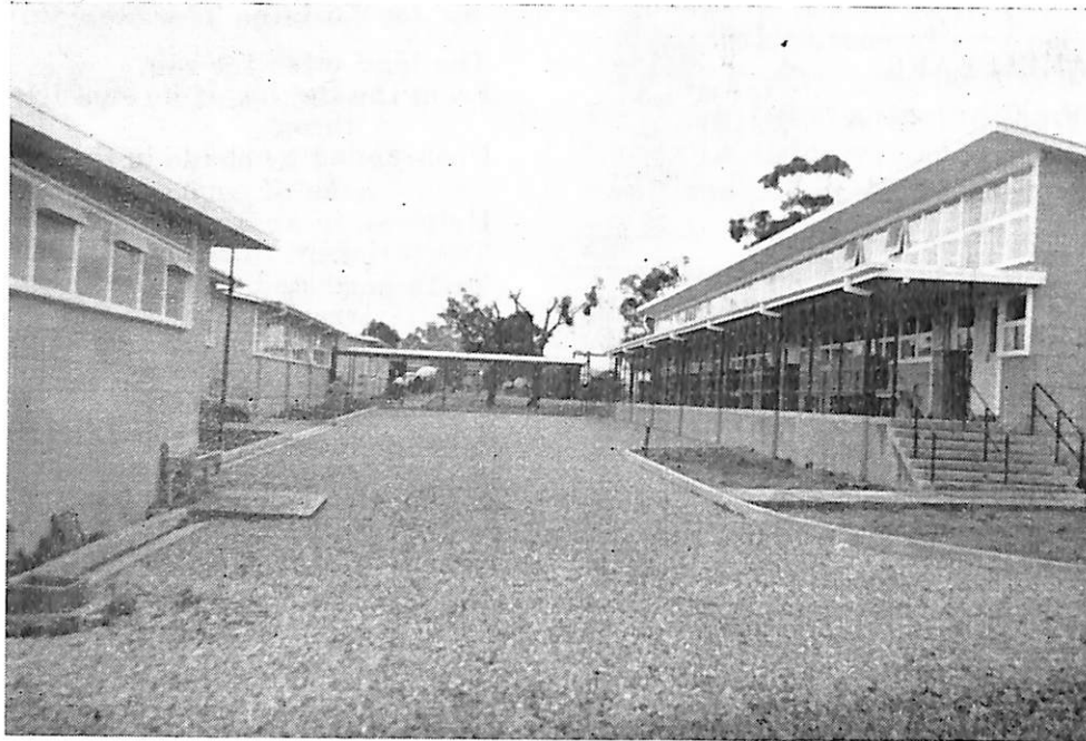
Manual Block prior to completion of the ground work.
