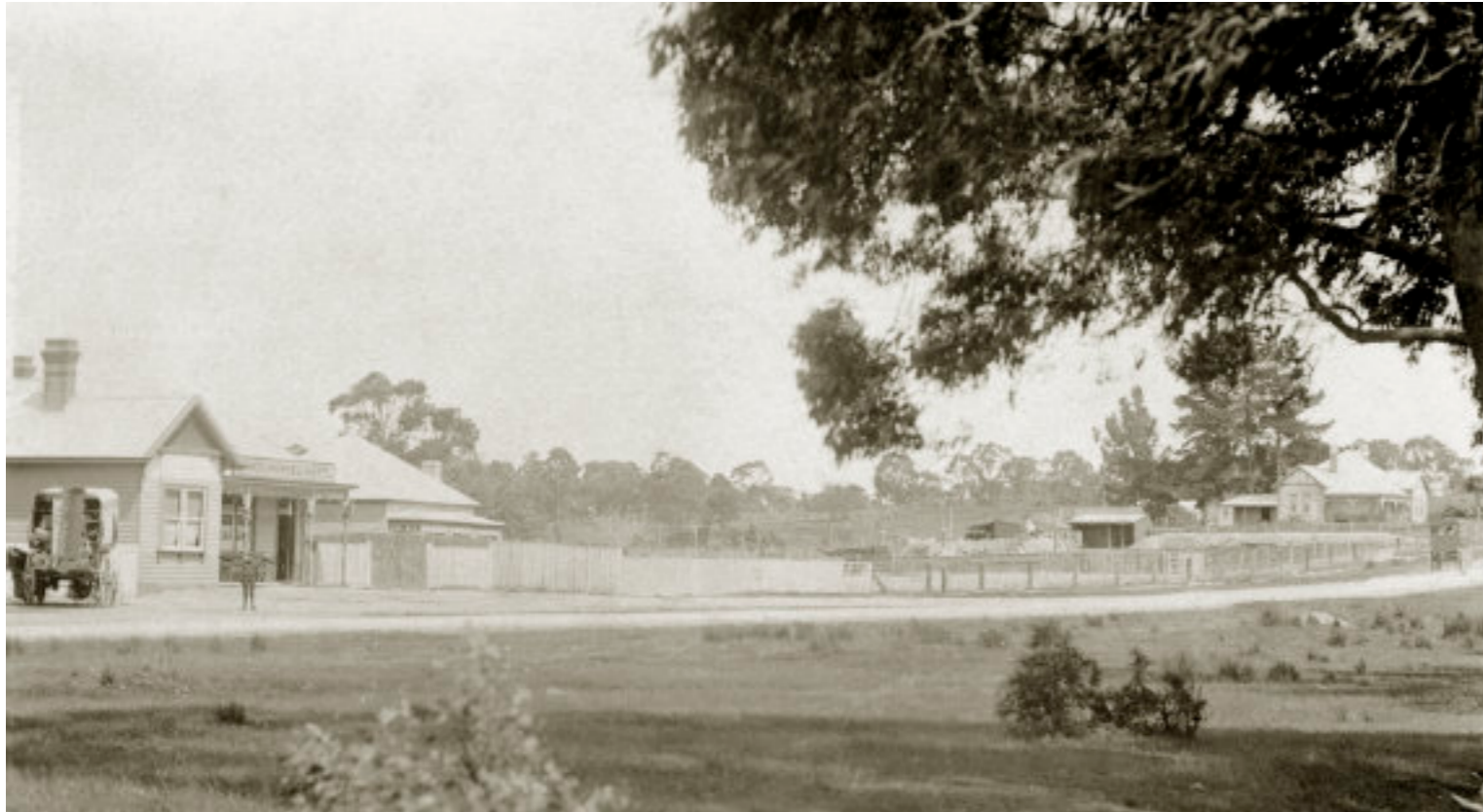
View of Whitehorse Road (now Maroondah Highway) in 1919 with the rebuilt Coach & Horses Hotel on the south side, following the fire of the original Log Cabin. Heatherdale Road is located on the top of the hill, past the large house on the right, in the west. Today, the Eastlink freeway bisects the photograph.
