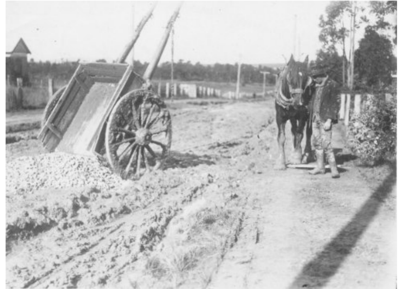
Sealing Wantirna Road by horse and cart (above). 1879 Shire Rate Book (below), showing some Ringwood pioneers.
