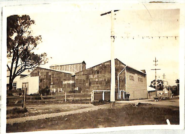
Temporary Repairs after Fire
