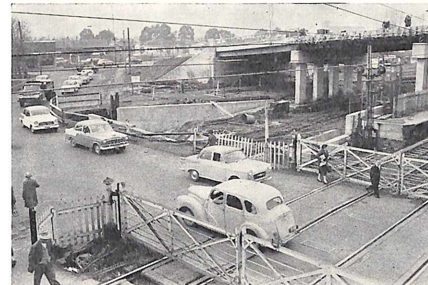
WELL-ADVANCED in construction is the new overpass at Sunshine; it will replace this busy level crossing at Hampshire Road. A single standard gauge track will be laid between the two piers (right). When the crossing is closed, road traffic will be diverted between the second pier and the abutment. (See News Letter , December 1960, Page 189, for an artist's conception of the completed overpass).
