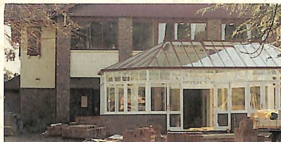
LATEST ADDITION - Wyreena's new conservatory in the final stages of construction.
