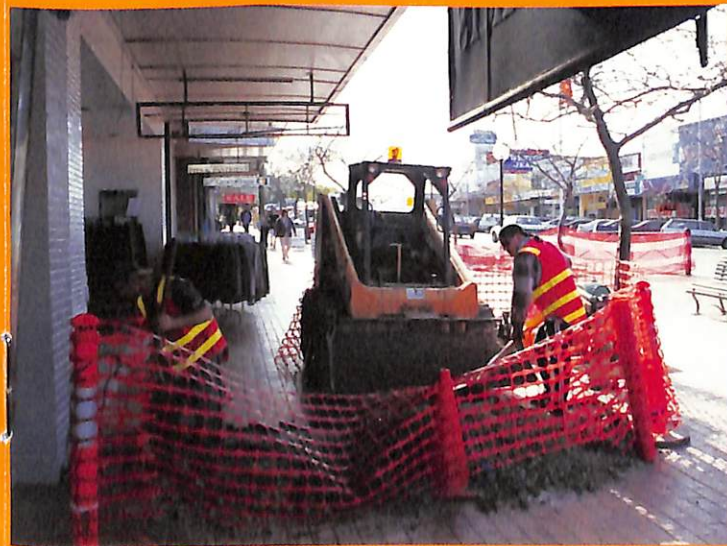
Undergrounding of power cables in Main Street is almost complete.
