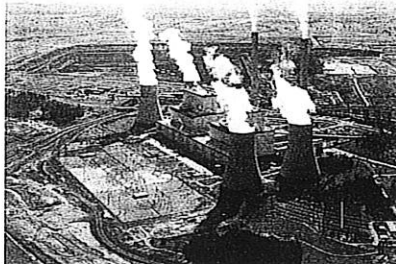
• The gigantic Loy Yang power station, south of Traralgon, completed in the mid 1980s.
