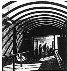
• Corridor roofs were originally glassed over.
