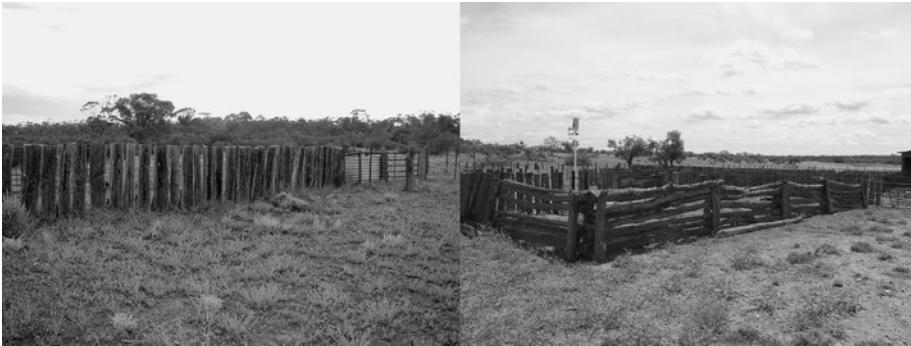
Figure 9. Paling fence and ‘double post-and-rail’ fence on Nanya Station. Source: M. Westbrooke January 2010.
