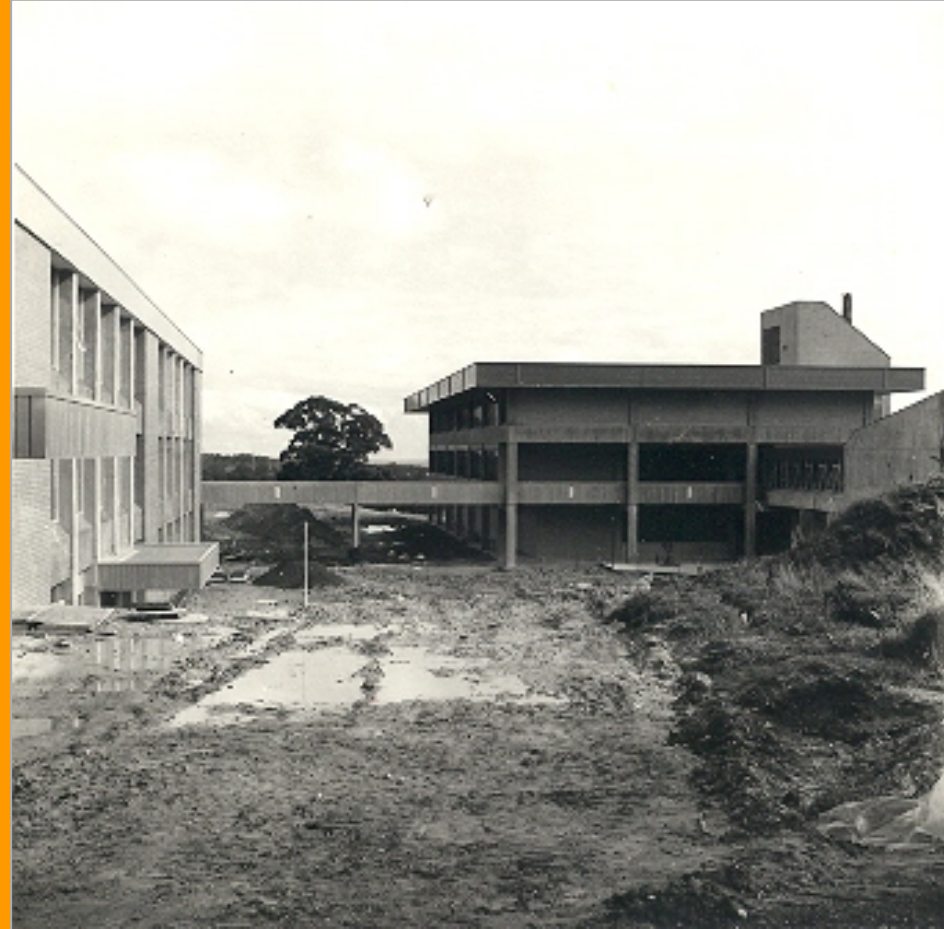
Muddy Courtyard, Mt Helen Library Under Construction, 1972
