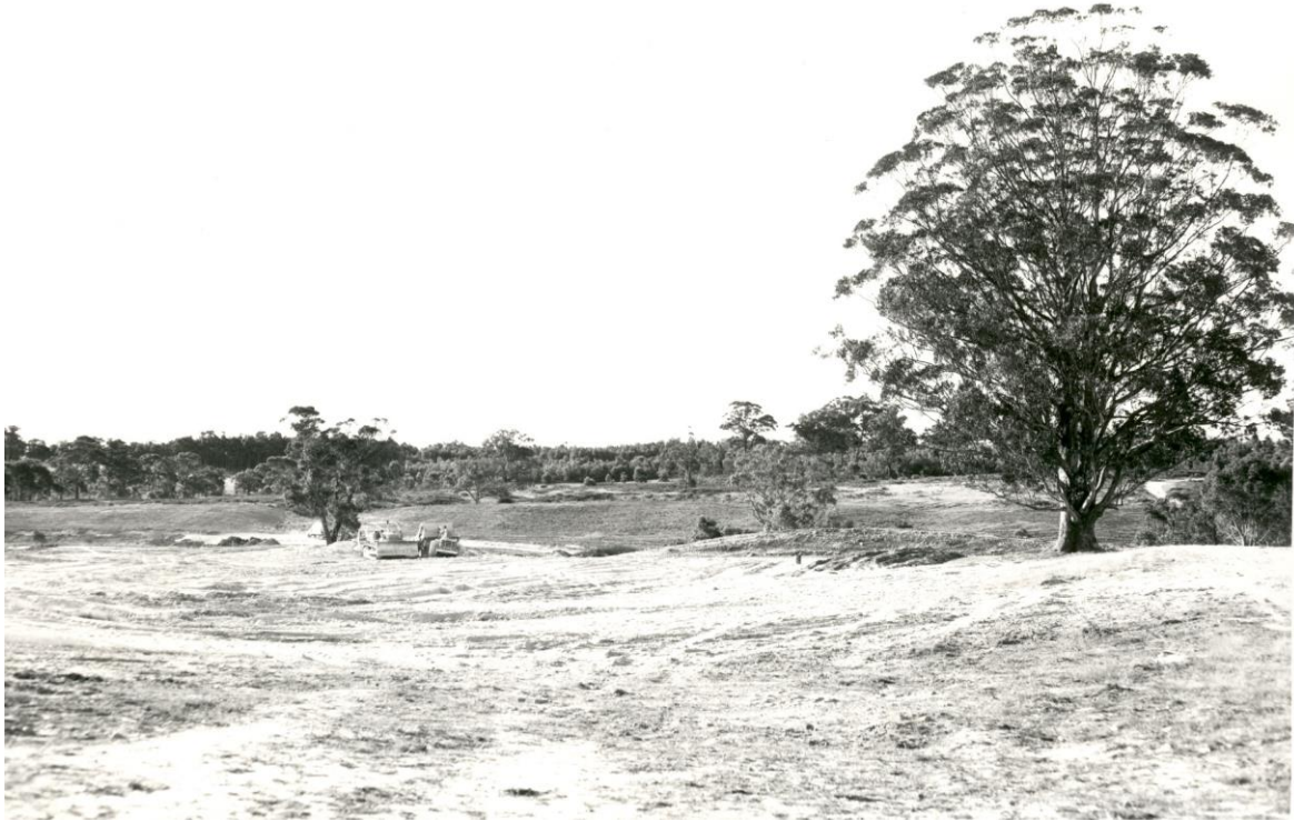
Preparing the site of the student amenities building, with Tree of Knowledge at right, Mt Helen Campus, c. 1971
