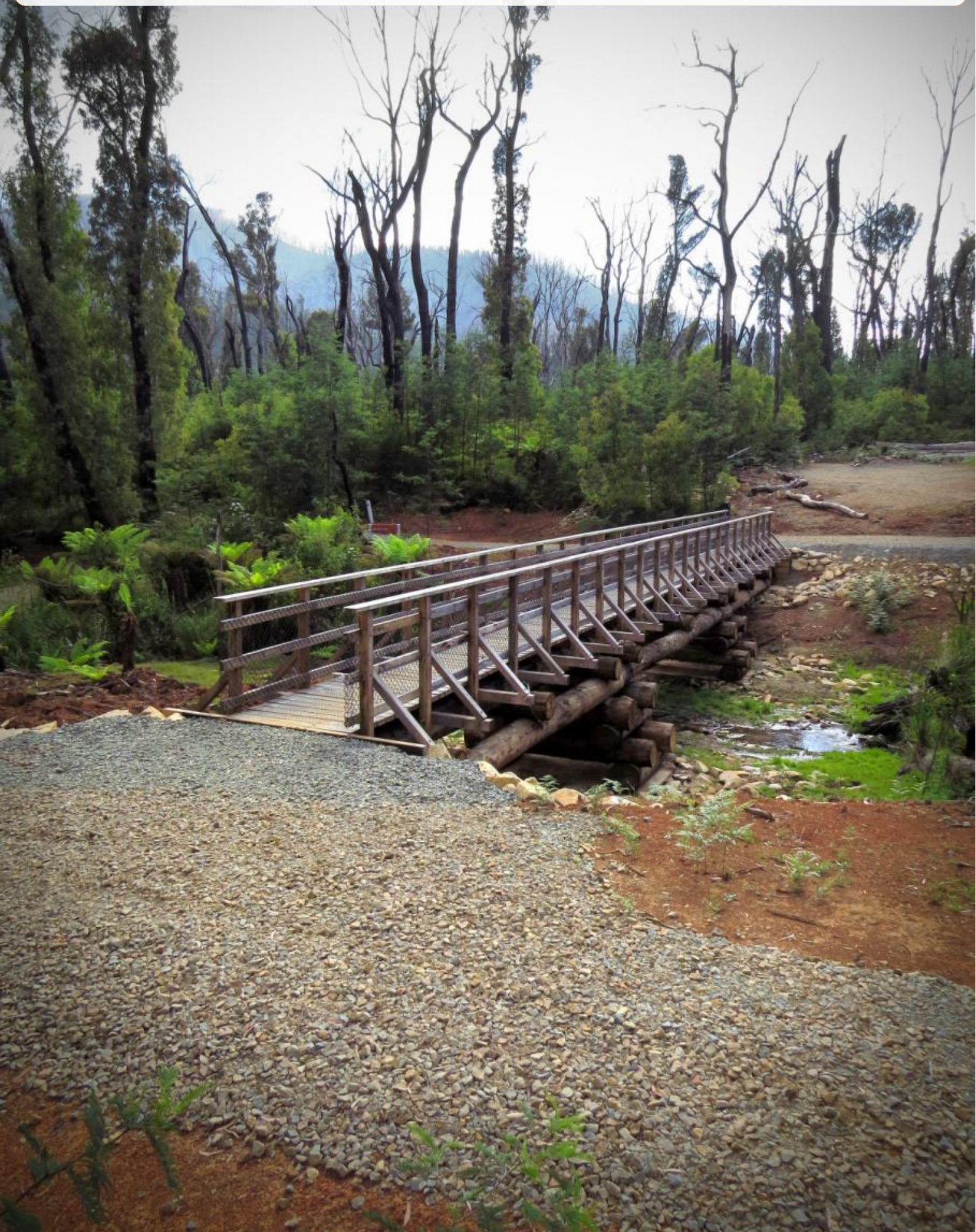
THE HISTORIC TIMBER TRAMWAY TRESTLE BRIDGE
