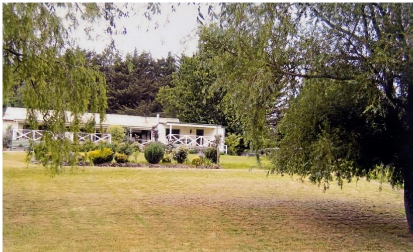
Rear view with the billiard room converted to B&B at the right end
