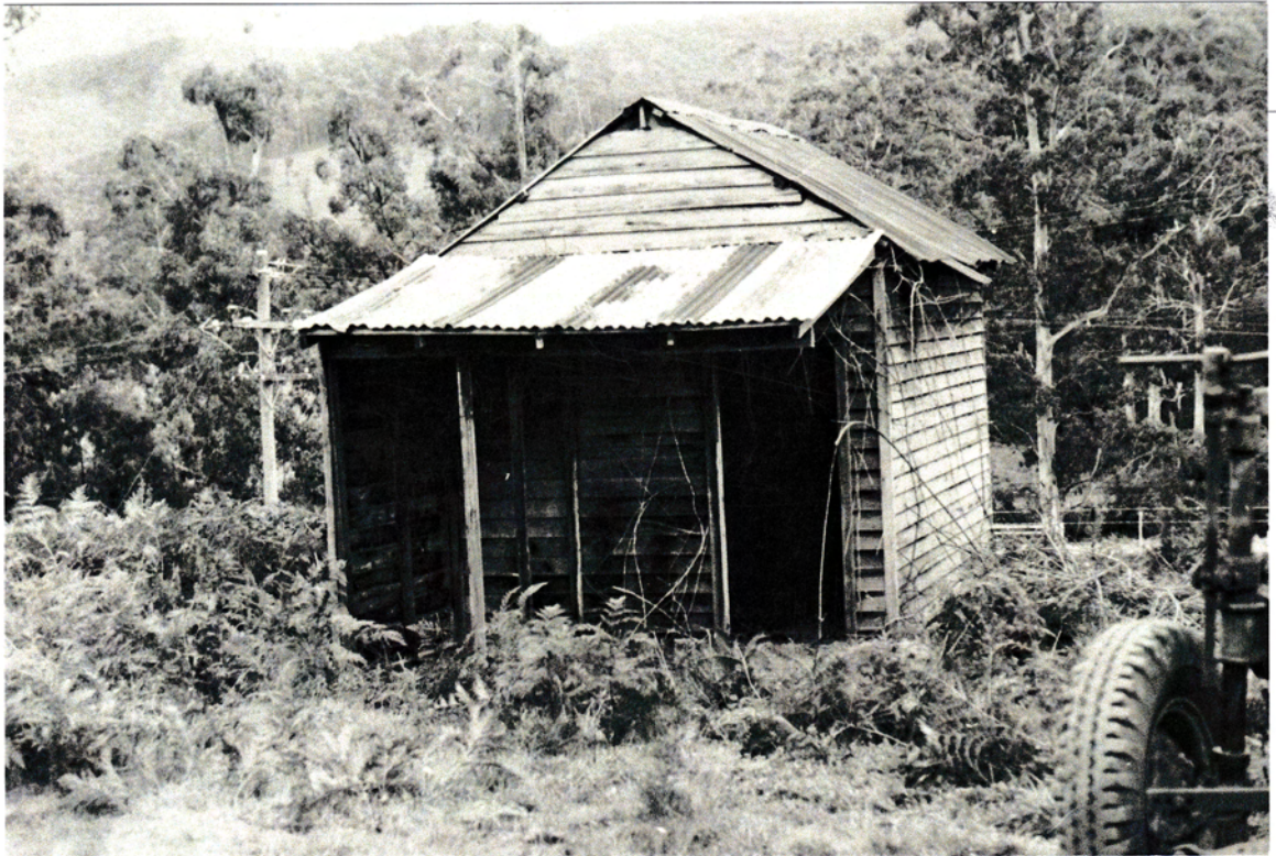
Photo 7: i, AN EXISTING BUILDING NEAR THE MAIN MILL
