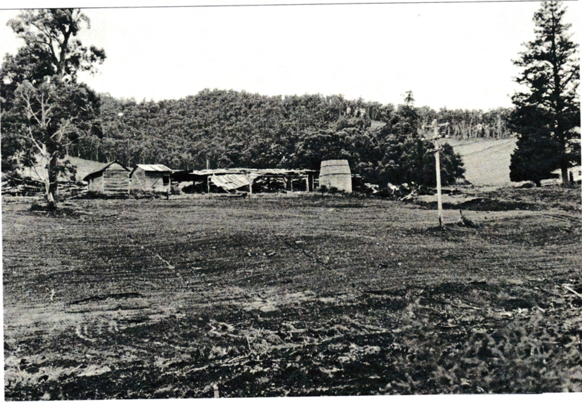
PHOTO 3: THE EXISTING MAIN MILL BUILDING.
