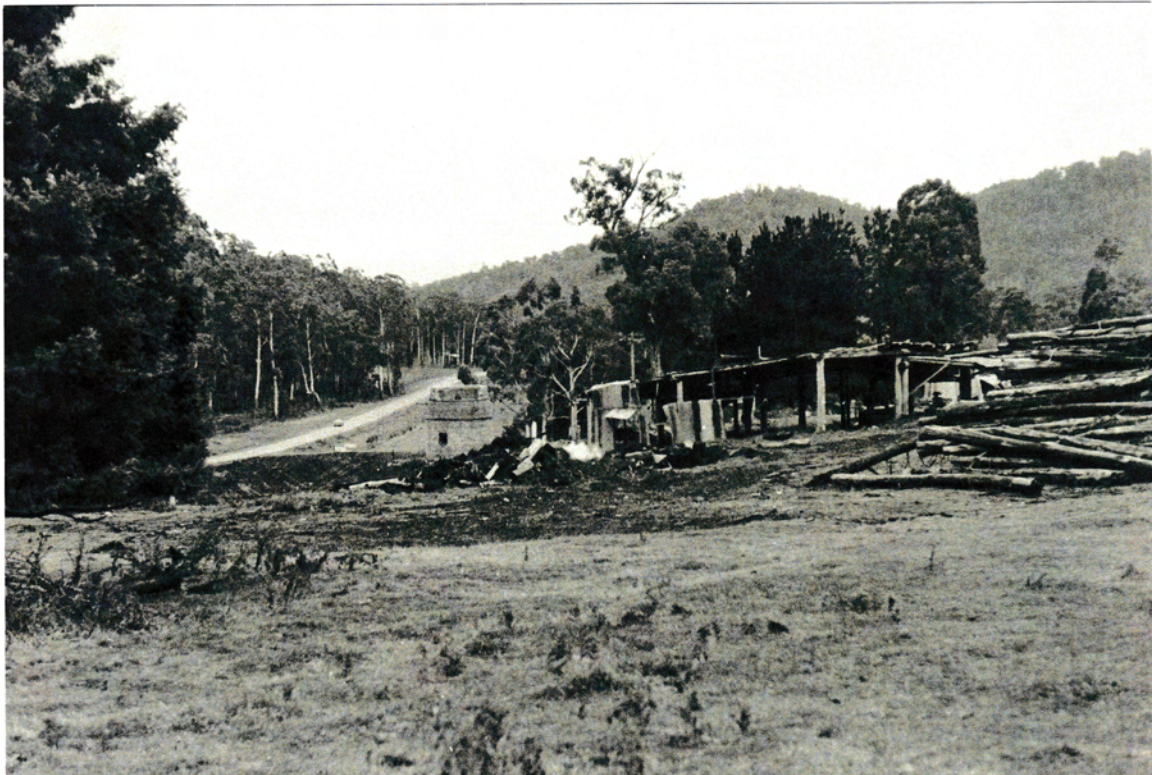
PHOTO 1: LOOKING NORTH. A VIEW OF THE REMAINS OF THE MAIN MILL BUILDING.
