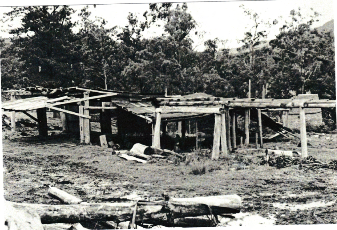
PHOTO 4: THE MAIN MILL LOOKING SOUTH WEST.
