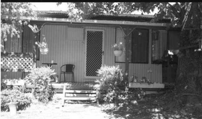
13 Hillside Avenue EILDON
