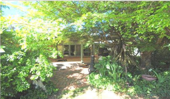
664 Goulburn Valley Highway THORNTON
