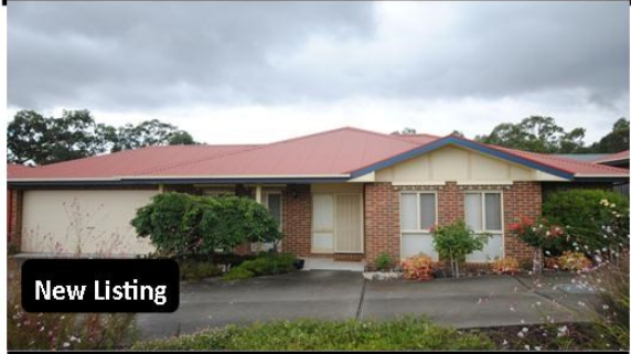
Unit 3/2 Thom Street ALEXANDRA
