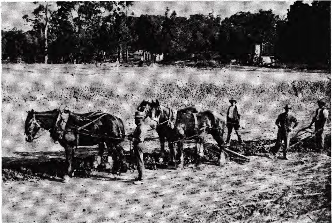
Building railway between Diamond Creek and Hurstbridge, 1910–1913.
