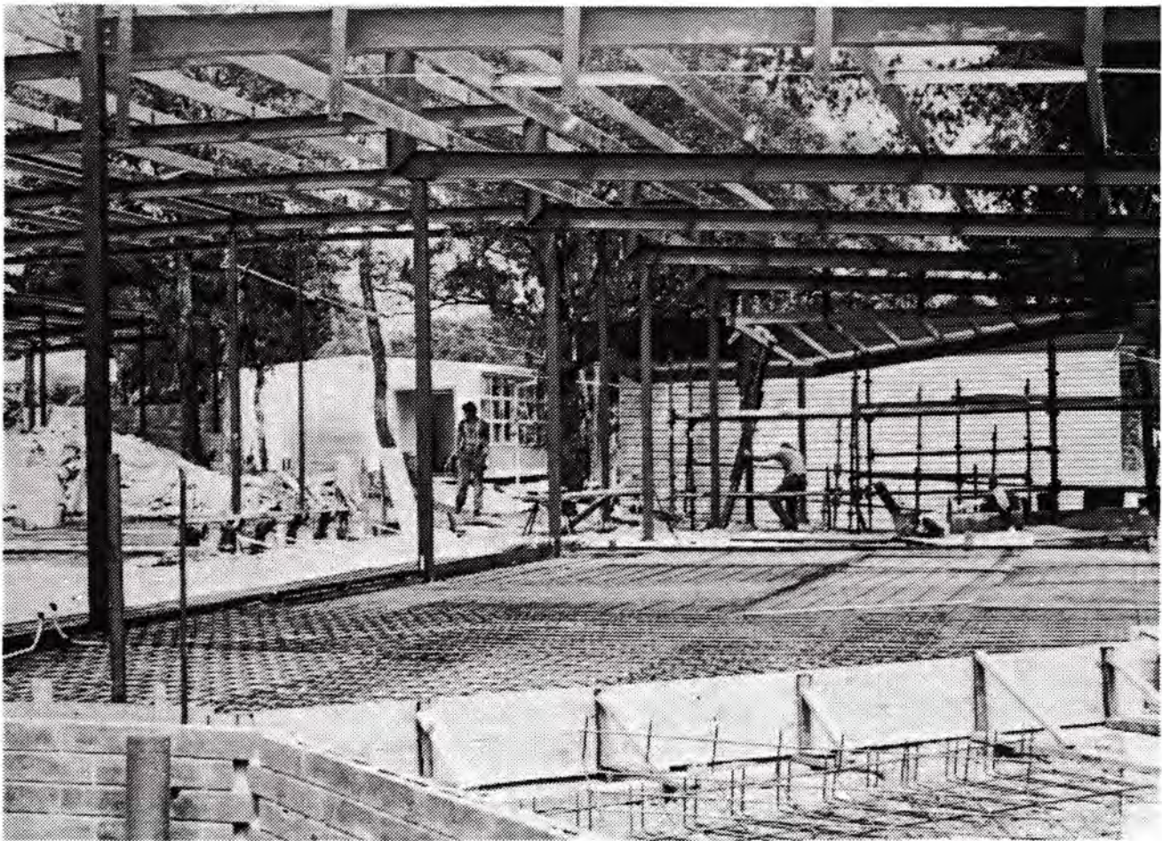
Re-building after 1976 fire.
