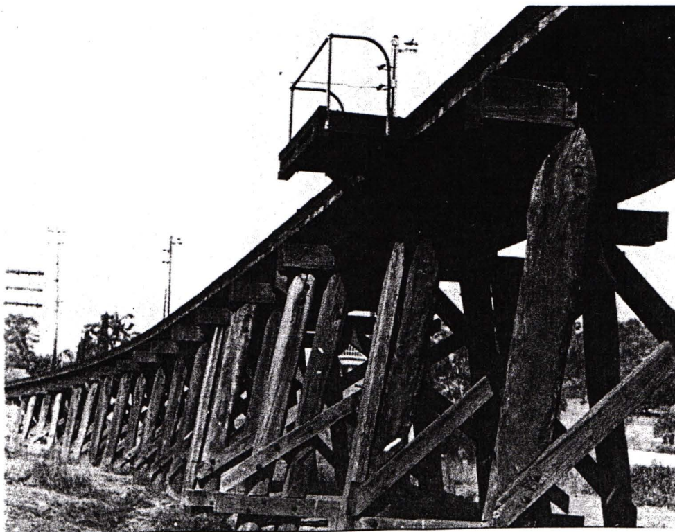
ELTHAM RAILWAY BRIDGE From the Society's collection of George Bell photographs from the 1960s
