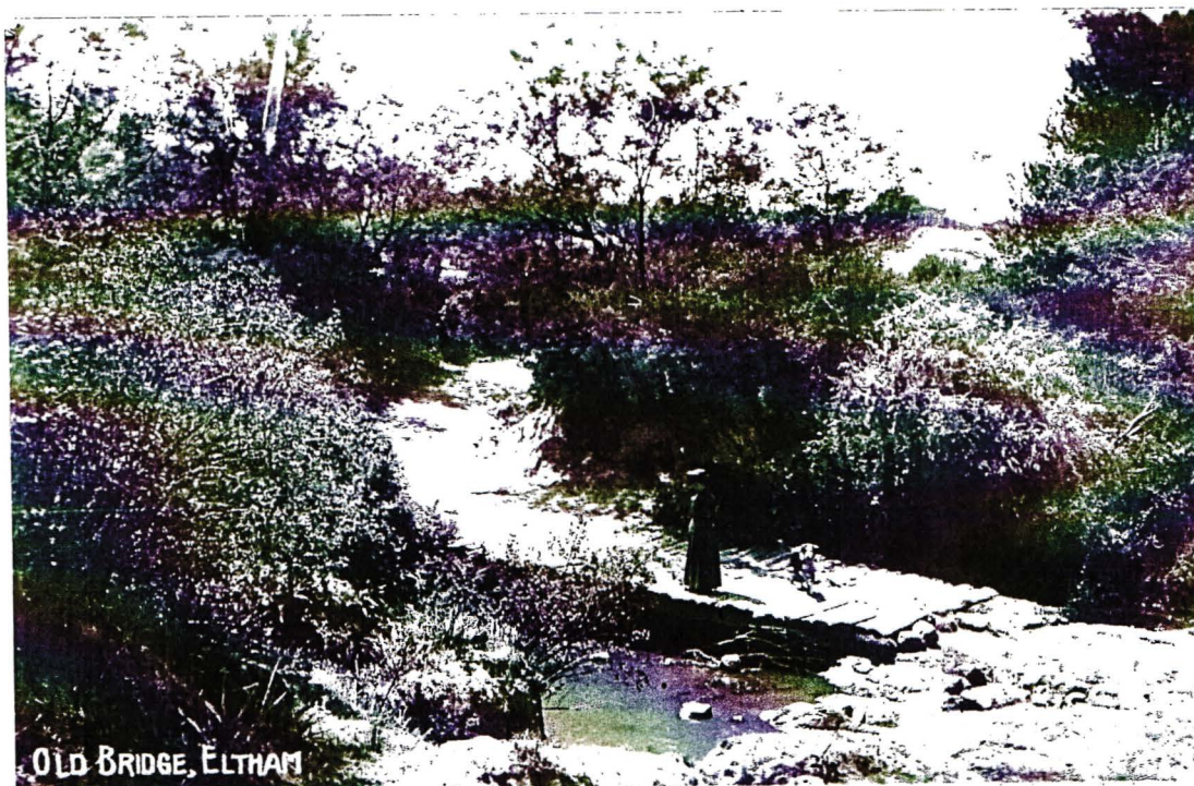
The old log girder bridge in Brougham Street
