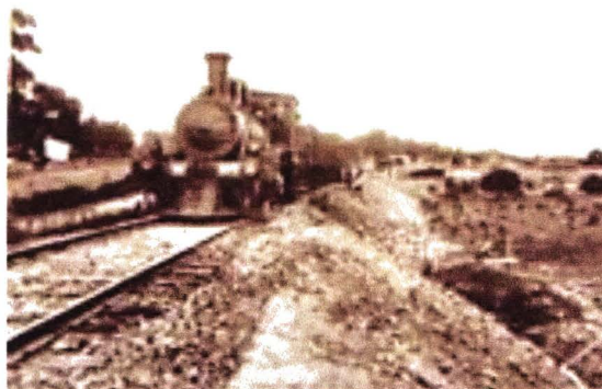
Eltham - Hurstbridge railway construction at Wattle Glen
