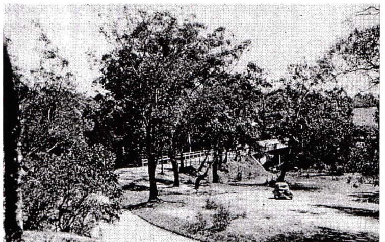
Main Road bridge over the Diamond Creek
