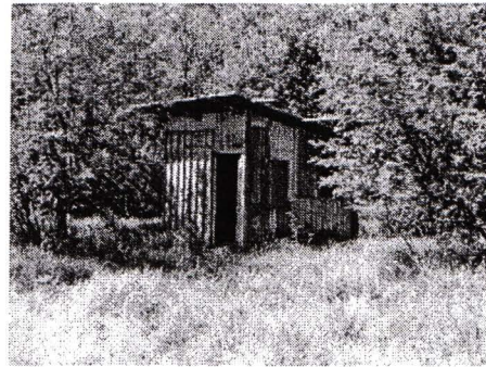
Former pump house on the land at 2 Bell Street, Eltham
