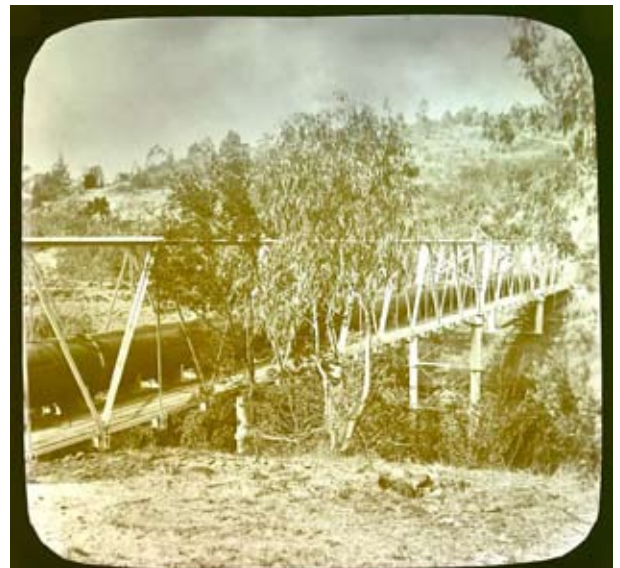
Early view of the Maroondah Aqueduct pipe bridge over the Plenty River at Greensborough, photographed by J H Henry, (National Library of Australia) from https://yallambie.wordpress.com/tag/greensborough/
