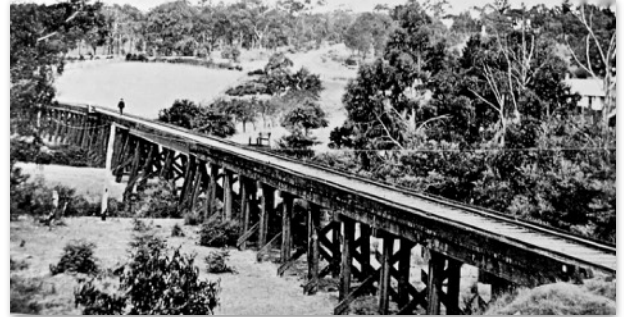
Eltham Trestle Bridge
