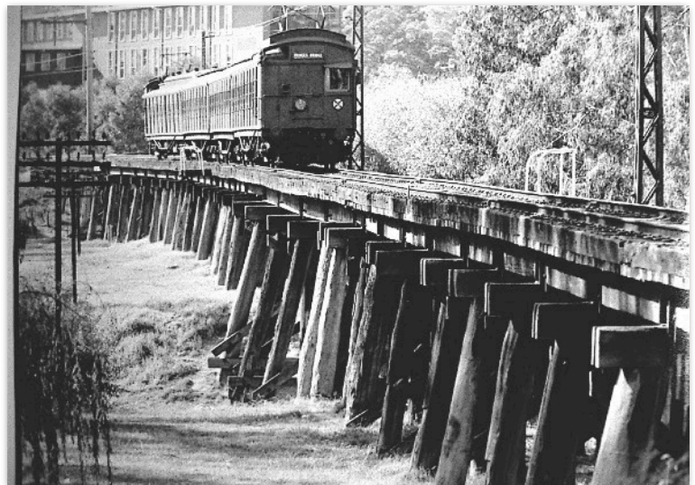
'Red Rattler' on Eltham Trestle Bridge
