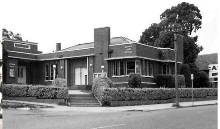
Eltham Shire Offices and Shire Hall
