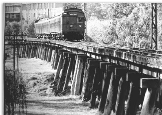
Eltham Trestle Bridge 1981 * Shire of Eltham Pioneers Collection
