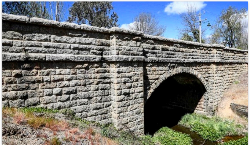
Commissioner’s Bridge, Yackandandah
