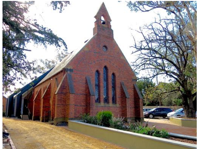
St Margaret's Church, Eltham Photograph by Jim Connor
